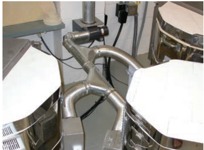
This shows several small kilns hooked up with one Vent-Sure using two Vent-Doublers. (Up to 20 cubic feet can be ventilated with one vent).
